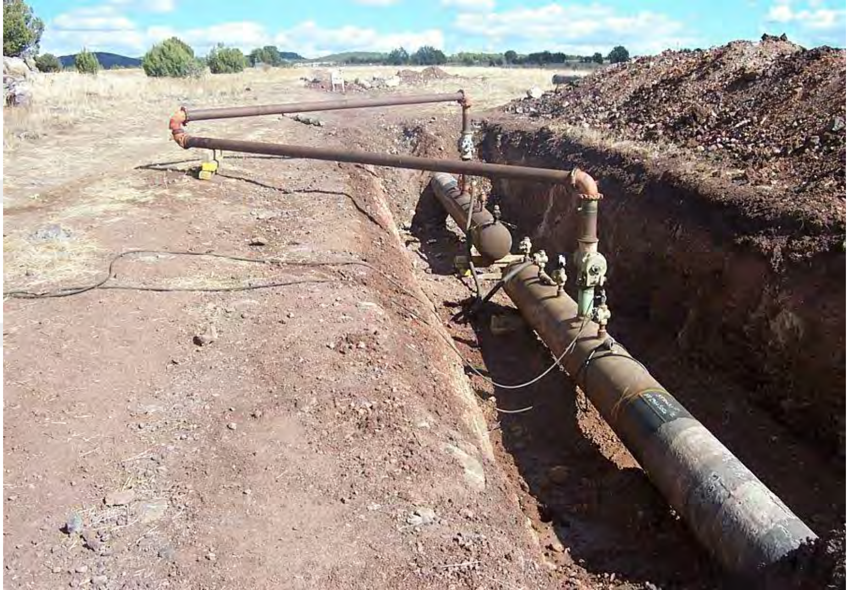
Jump-Over Line Between Two Test Sections
