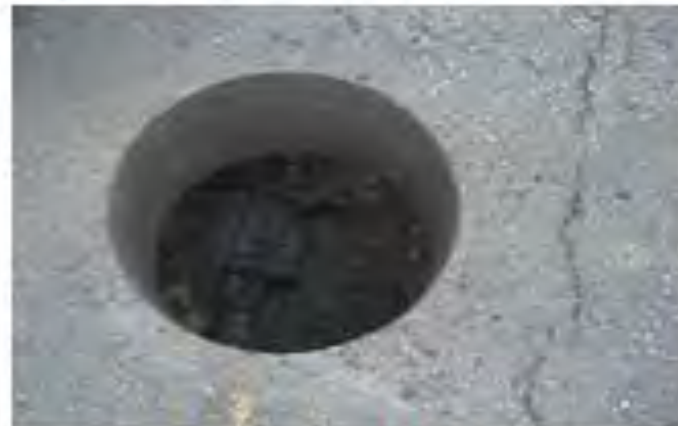
Flange Joint located by MJL
